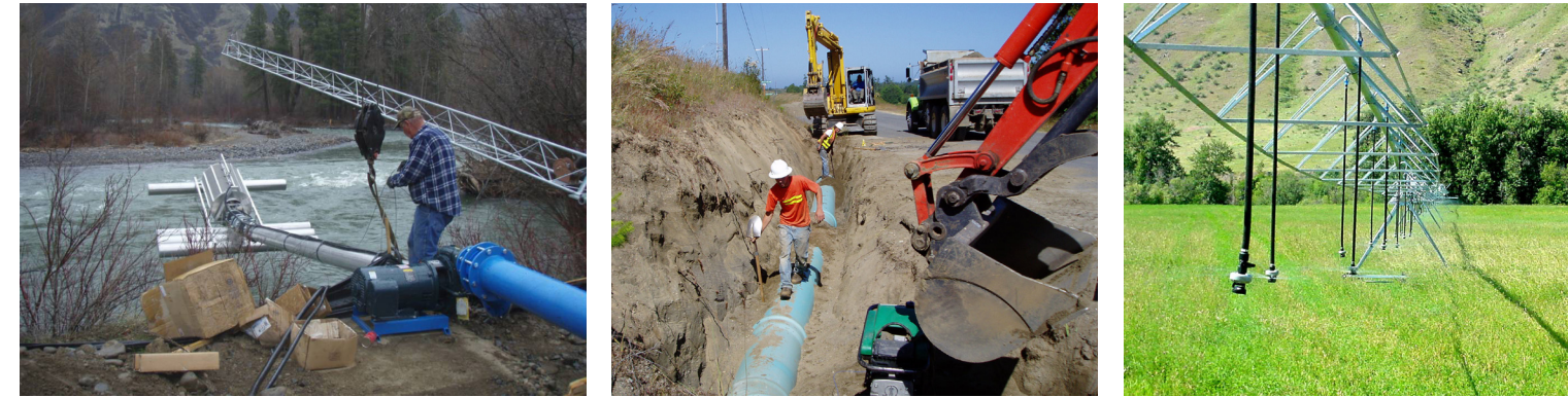
Left: Fish screens are cost-eligible and required on IEGP projects. Fish screens protect juvenile fish from water diversions, such as irrigation pump intakes. Middle: Converting open ditch irrigation systems to pipeline systems not only saves water, it also helps prevent polluted runoff from impairing water quality. Right: Many IEGP projects fund center pivot systems, which are one of the most efficient and effective irrigation system types. They help save water, energy, and time.
